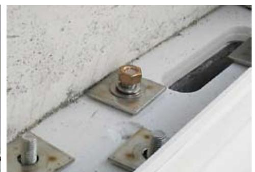
Install flat plate, flat washer, lock washer and SS nut.
