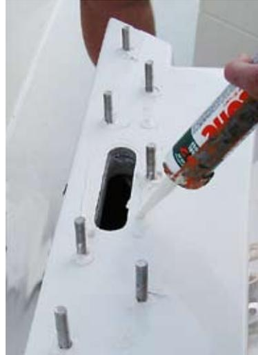
Install sealant around studs and openings
