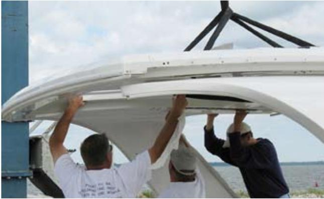
Carefully line up top with sides. It might be necessary to start a couple of bolts on one side first and then line up other side.
